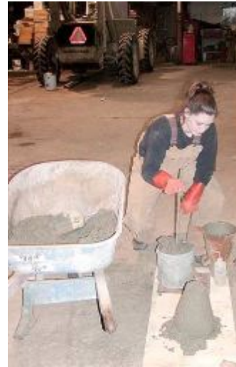
Nicole Lupro, a technician for Alaska Concrete Casting, tests for slump and air content during a cold-weather concrete demonstration held in Juneau in early February. PHOTO Courtesy of SpringBoard
